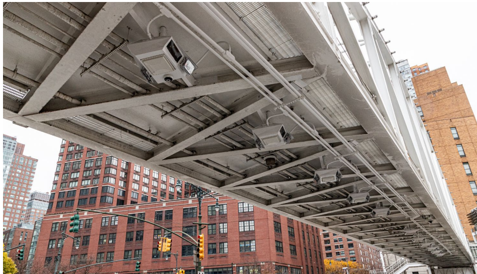
West Side Highway at Chambers Street, Tribeca Pedestrian Bridge
