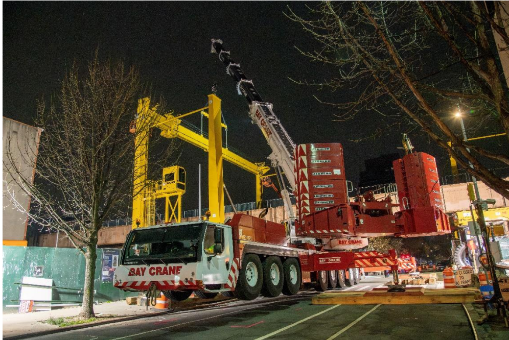
Overnight gantry construction
