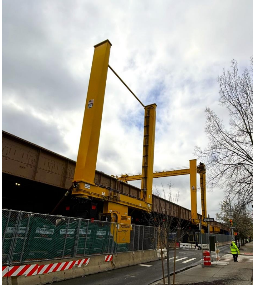
Gantry with one of four top beams in place
