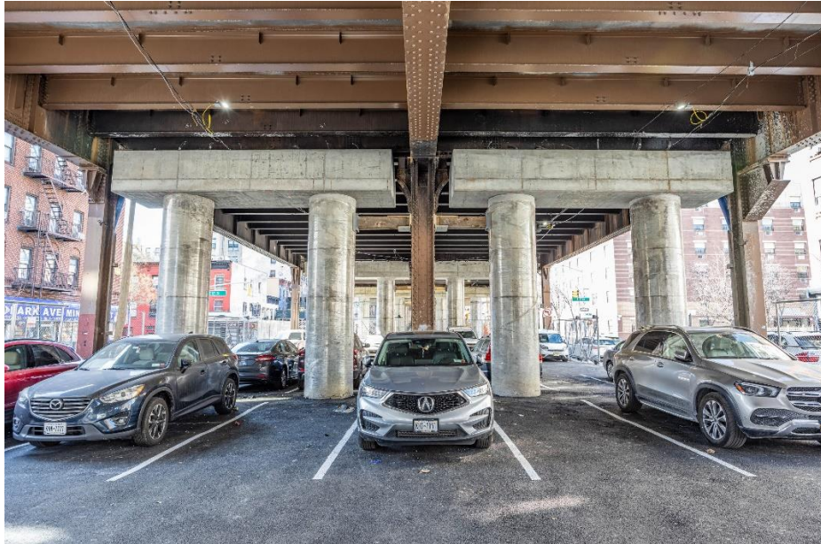
Completed columns at Lot 7 between E. 117 th and E. 118 th Streets
