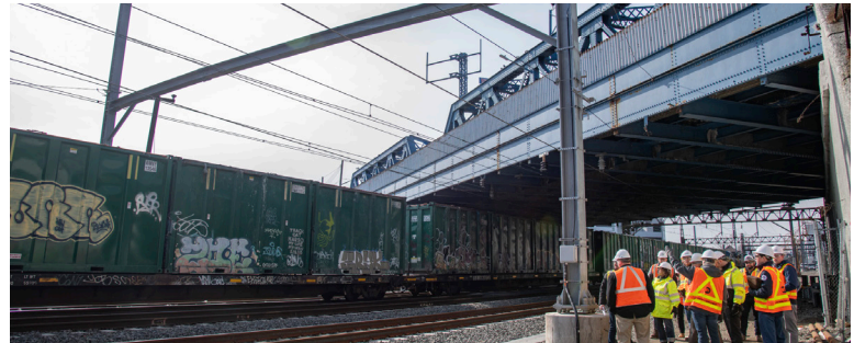
A completed portal at Leggett Interlocking. February 2024.
