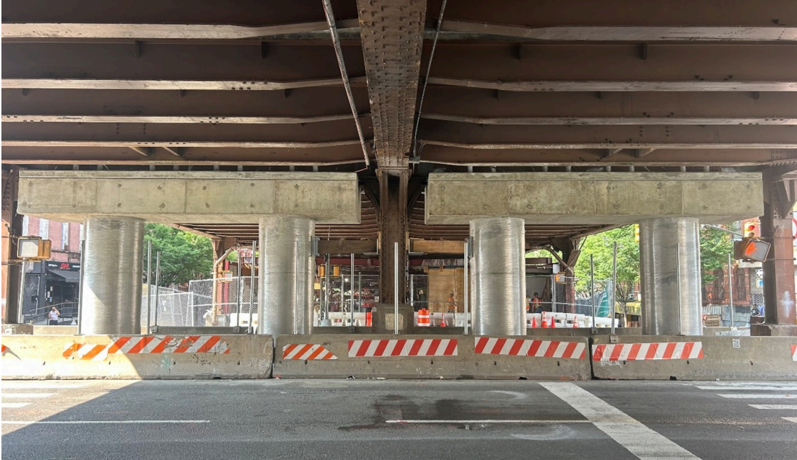
New Foundations, columns and pier caps at East 116th Street
