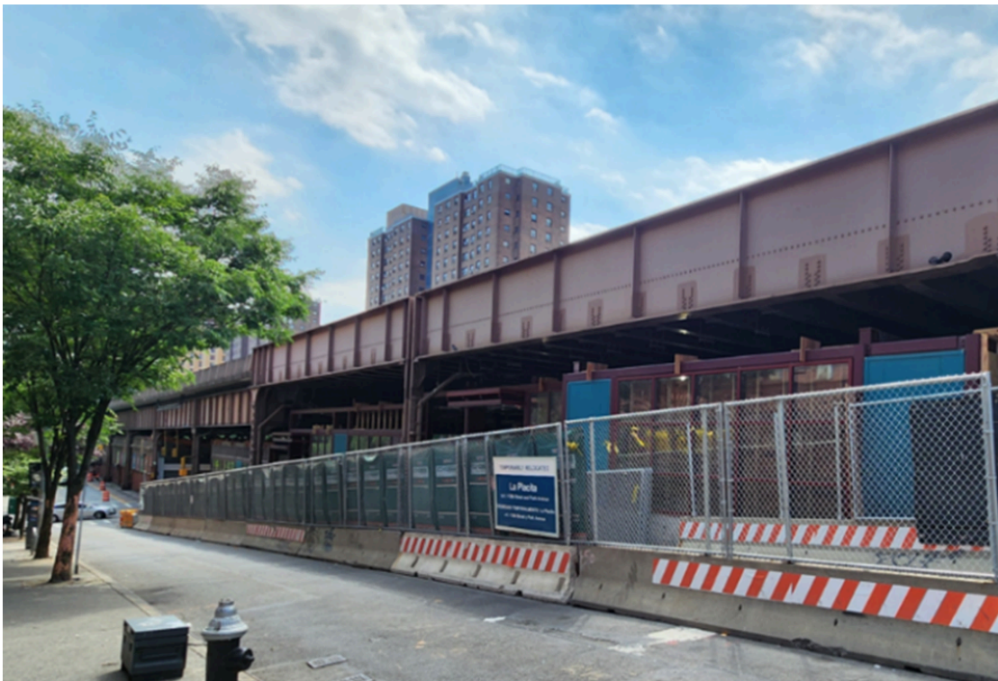
Temporary work zone protection around La Placita
