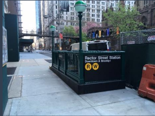
Rector Street Station Stairs completed (SBMP)
